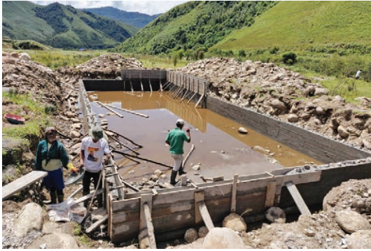
Fig. 65: (a) & (b) Trout raceways under construction at selected sites, Menchukha
